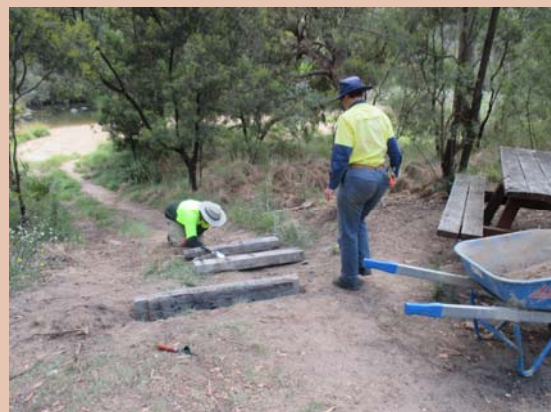
Bush Regenerators construct new steps onto the river bed to facilitate pedestrian access and hinder access by vehicles.
