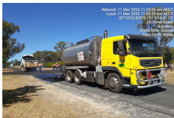
Image (above): Bitumen resealing in Bundarra
