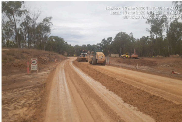
Image (above): Laura Creek roadworks preparing road base and the completed project with extended guardrail.
