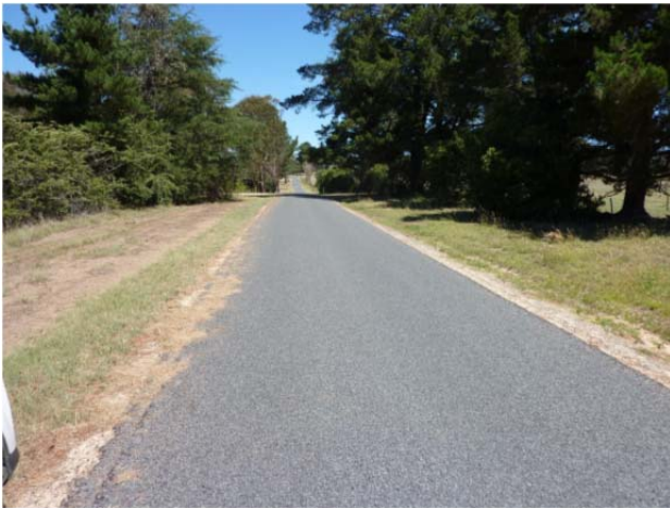
Sealed Road – Condition 1 (Eastern Avenue)
