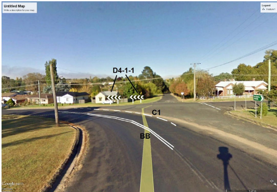
Figure 3 - Mark-up provided by TfNSW (hazard markers installed. Line marking programmed)
