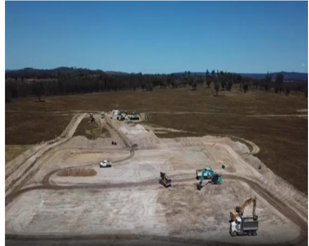
Ledonne Construction of the Bundarra Sewerage Treatment Plant in February 2021. equipment.
